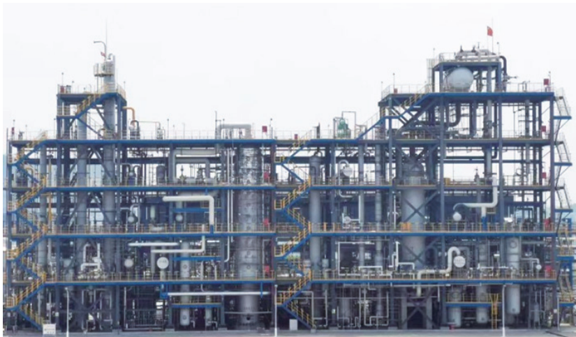
A 50,000-ton/year industrial unit for converting ethylene into isopropanol.
